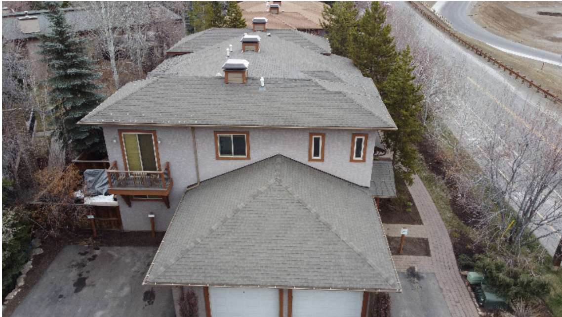
Building Exterior - Roof, Asphalt Shingle
