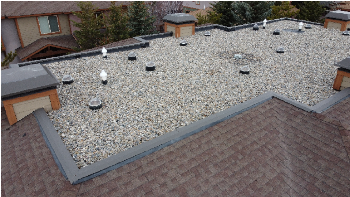
Building Exterior - Roof, Low Slope, Membrane w/ Ballast
